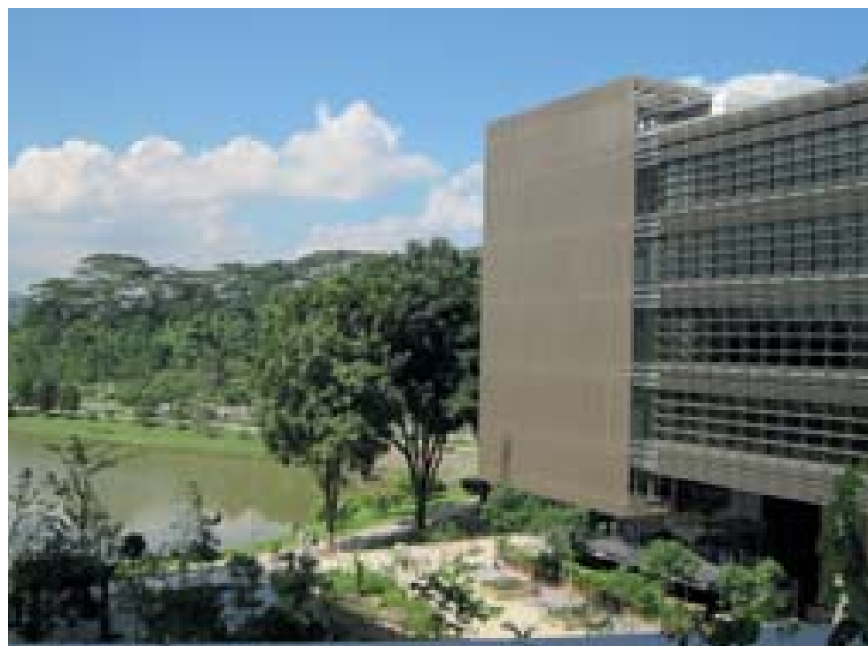
Vertical fins and jalousies at KTPH funnel air into a building to cool it. Greenery encourages local wildlife onto hospital grounds.
