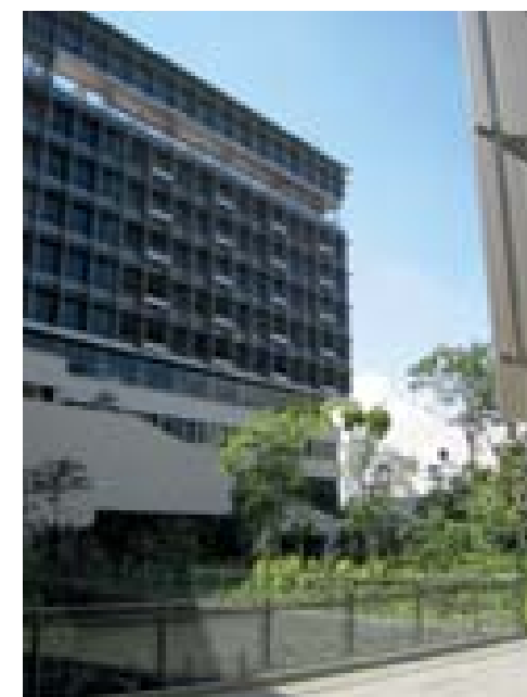
This 10-storey building houses the eight naturally ventilated public wards at KTPH.
